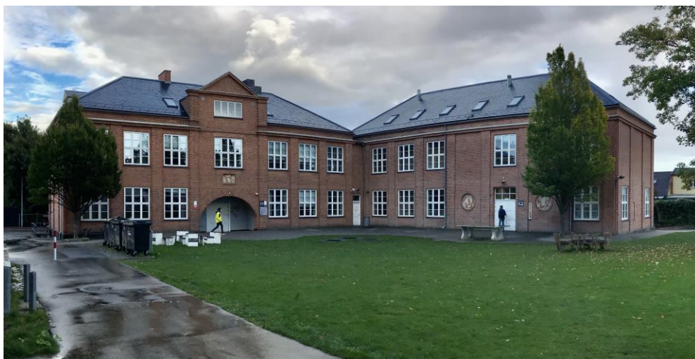
Figure 5-2. The Danish school building in which an MPC was installed and controlled the indoor air temperature.
